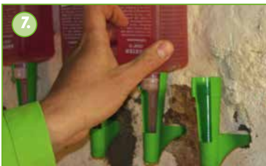
7. The Capillary Rod must not be prewetted anymore. The nozzles of the cartridges sit directly on the capillary rod providing material to be soaked in.
