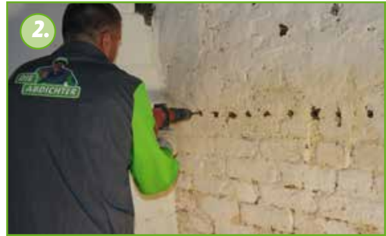
2. Boreholes are drilled into the interior walls at a distance of 10 cm from each other (wall thickness 45 cm) up to a depth of 40 cm.
