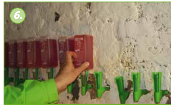
6. The KÖSTER Crisin 76 Concentrate cartridges are installed.
