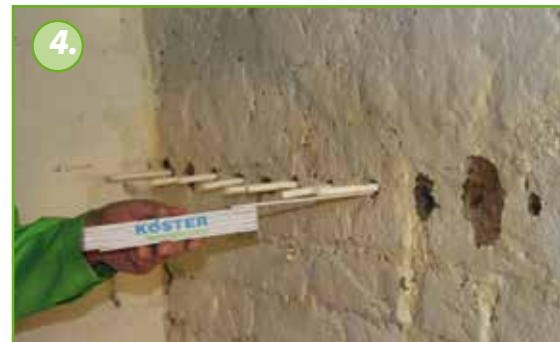
4. KÖSTER Capillary Rods are installed so that they protrude 7 cm from the borehole.
