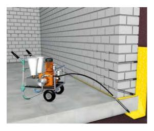
In cases where an existing basement is leaking and the soil surrounding the building cannot be excavated, the waterproofing has to be done from the inside. With KÖSTER PUR Gel it is possible to create an exterior waterproofing layer
