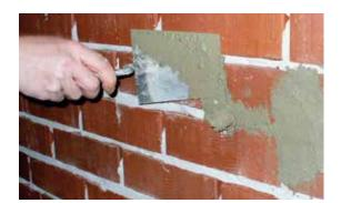
All holes wider or deeper than 5 mm have to be filled using KÖSTER WP Mortar. Gravel nests, break outs, construction joints and other areas which are susceptible to leaking or which are difficult to coat must be opened up and filled with KÖSTER WP Mortar.
