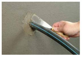
The pipe penetration is now waterproofed. In order to protect the waterproofing the area around the pipe or cable is plugged with KÖSTER KB-Fix 5.
