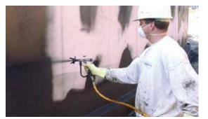
KÖSTER Deuxan<sup>®</sup> Professional is similar to KÖSTER Deuxan<sup>®</sup> 2C but specifically designed for spray application with a suitable spraying device. Spray application provides a very high productivity which makes it attractive for professional contractors and for larger objects. It requires knowledge of the pump and the spraying process. The spraying equipment has to be tested and fine tuned before commencing work.
