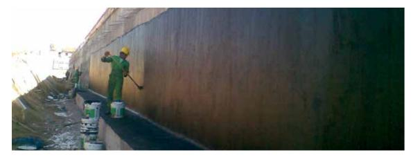
Below grade waterproofing is the core discipline of any waterproofing specialist. About 80% of the damages in construction are directly or indirectly linked to problems caused by moisture. In contrast, a reliable protection against moisture can typically be achieved for less than 5% of the total construction cost. Waterproofing does not only protect buildings but investments. That is why a high quality waterproofing is so important.
