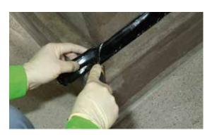
Fillets can be made of either KÖSTER WP Mortar or alternatively with the cold self-adhesive KÖSTER KSK Triangular Ribbon.
