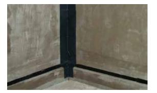
After that, the membrane is applied to inside and outside corners.
