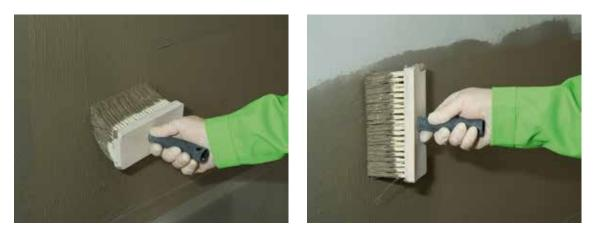
KÖSTER NB 1 Grey is applied using a coarse brush. Make sure to brush up and down as well as left and right in order to close all pinholes.
