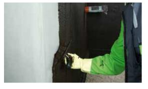
The first layer of KÖSTER Deuxan<sup>®</sup> 2C is applied, in this case by trowel. Surface profiles and unevenness up to a depth of max. 5 mm are filled with a scraped layer of KÖSTER Deuxan<sup>®</sup> 2C.
