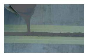
of the construction member without causing any damage. Normal Construction joints up to 35 mm can be sealed with KÖSTER Joint Sealant FS. For wider joints (like dilation joints) we recommend KÖSTER Joint Tapes.
