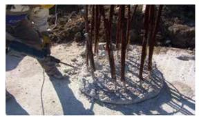
Removing protrusions, cleaning the pile head
