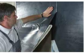
*The area is waterproofed with the membrane. Membranes must overlap by approx. 10 cm.*
