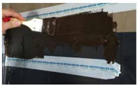
The edges of the membrane are sealed with KÖSTER KBE Liquid Film.
