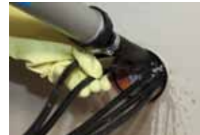
2. ... pipe is sealed...
