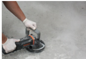
1. Substrate preparation
