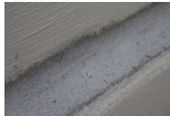
2. Fillet installed with KÖSTER Repair Mortar
